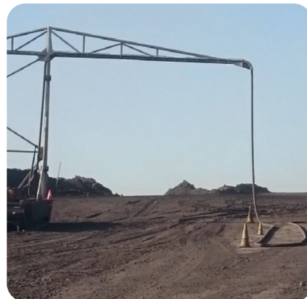
Cable suspended above guideways
